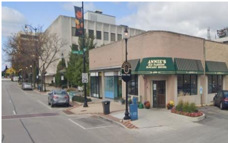
Site of proposed Hotel/Garage Project
